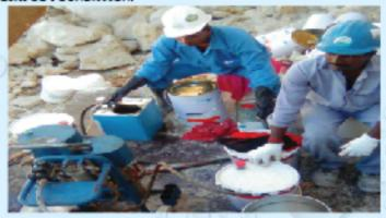
INJECTION TO STOP LEAK FOR SHORING (SECANT) PILES
