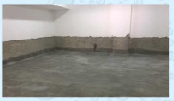
CONCRETE REPAIRS AND GROUTING TO FIRE EFFECTED CEILING AREAS PROJECT: TAMWELL TOWER AT JUMEIRAH LAKE TOWERS, DUBAI. MAIN CONTRACTOR: M/S ALEC CONTRACTING.
