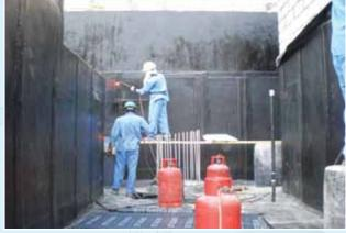
3 Basement Pile Foundation - Bitumen WP System | 3B+G+40 Tower at Jumeirah Lake Tower - Dubai
