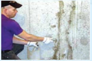
Crack and Leak Injection | Basement of Head Office Building | National Bank of Abu Dhabi
